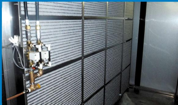
UC-EU1 type installed into AHU.
